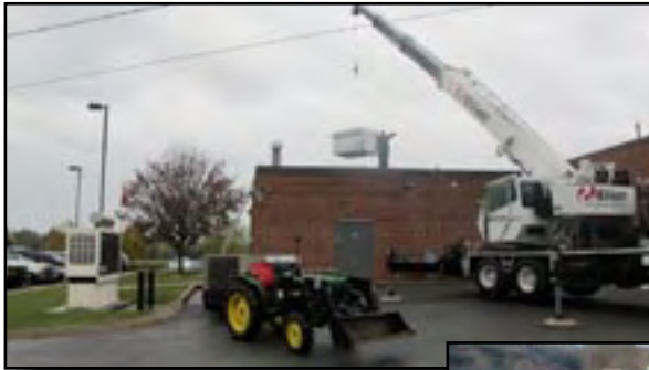
Construction gets underway for the Cannon County jail.
